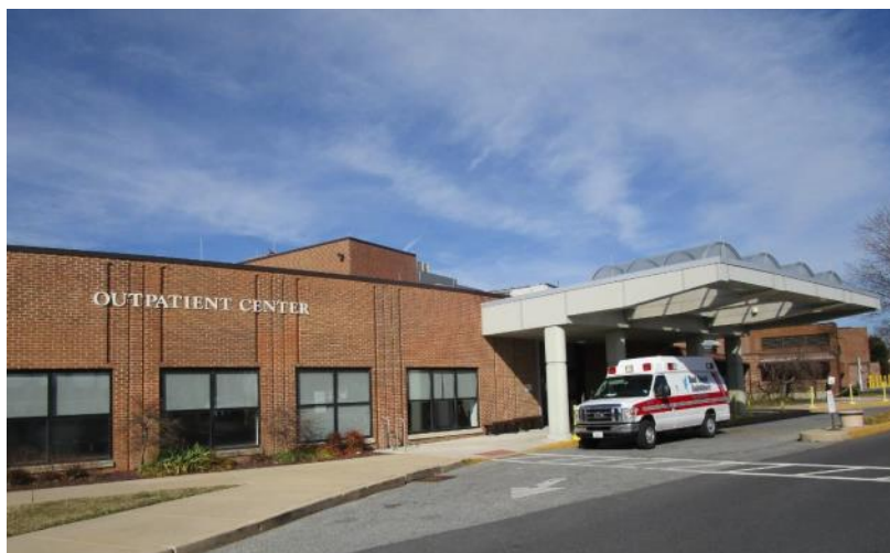
Bayhealth Outpatient Renovations
