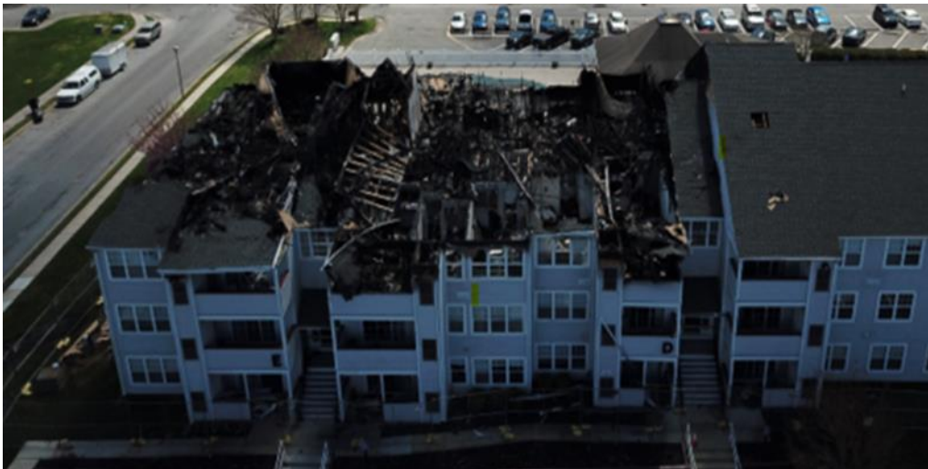
Baytree Apartments Building D/E after fire damage. Date of photo is 4/27/2020.
